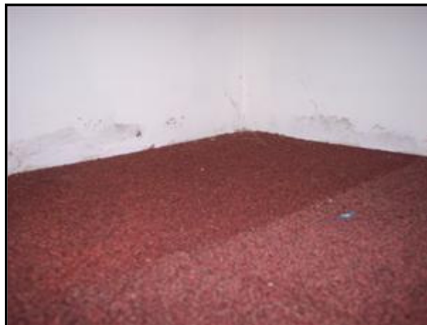
3.0 Picture 1 Water damaged drywall
