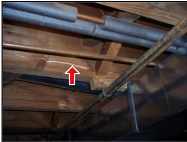
3.3 Picture 3 Cracked floor joist in basement
