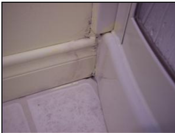
8.7 Picture 3 Evidence of leakage at shower stall
