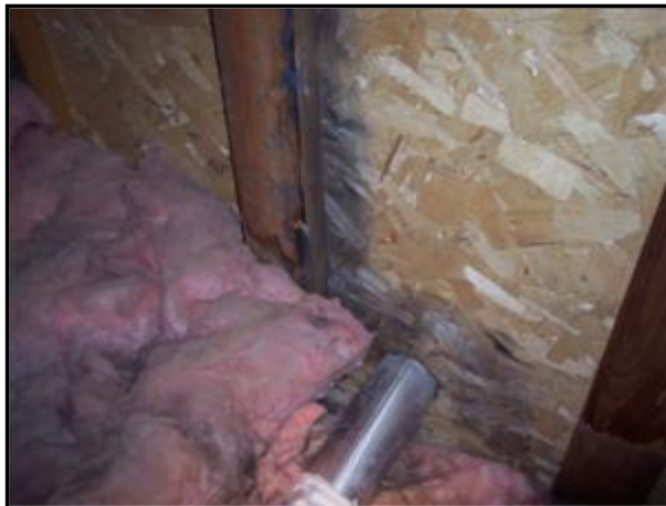
1.4 Picture 1 Water staining at exhaust duct penetration in attic
