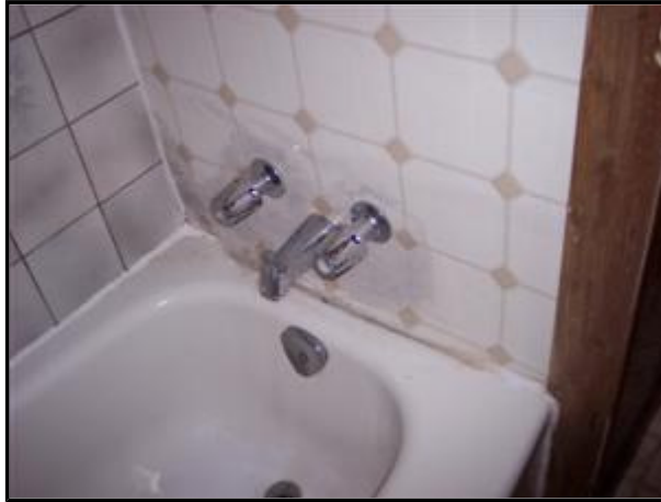
8.7 Picture 1 Water damaged tub surround
