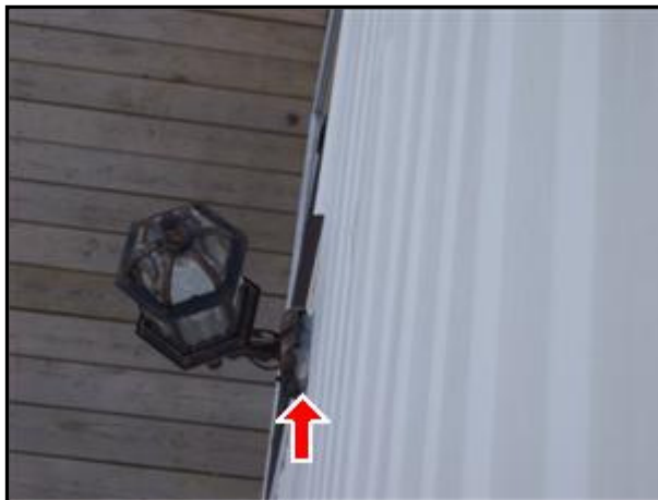
6.3 Picture 4 Exterior light fixture
