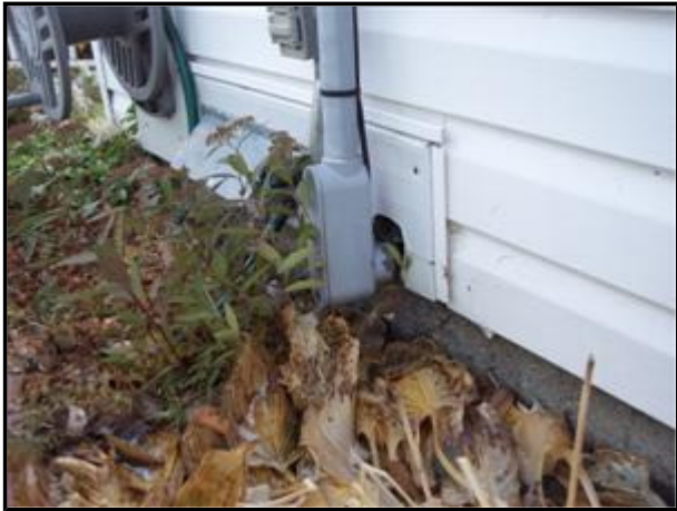
6.0 Picture 2 Broken conduit at service entry
