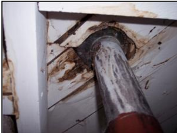
3.3 Picture 1 Water damaged subfloor under toilet
