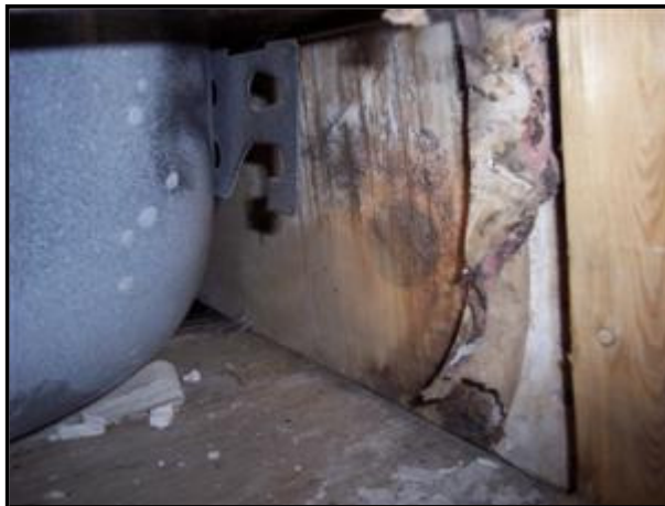
8.7 Picture 2 Moldy drywall behind tub
