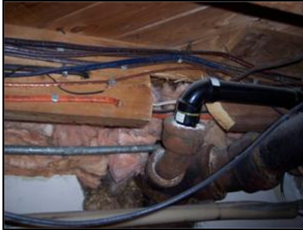
3.3 Picture 2 Damaged joist at east side of basement
