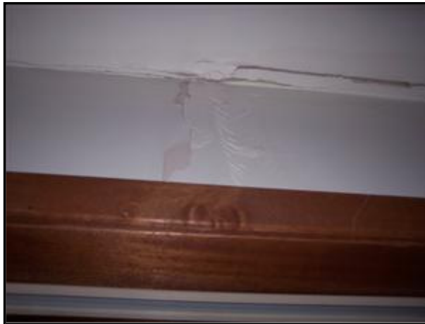
8.0 Picture 1 Water damage above living room window
