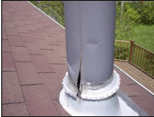
1.2 Picture 1 Damaged chimney
