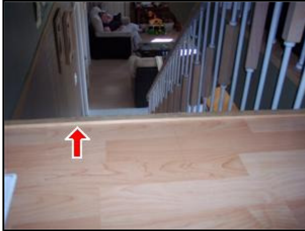
8.3 Picture 1 Trip hazard at top of stairs
