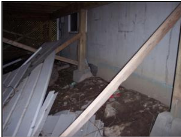
2.5 Picture 2 Foundation support for deck
