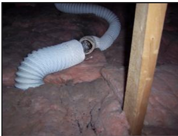
9.4 Picture 1 Bathroom exhaust fan duct in attic
