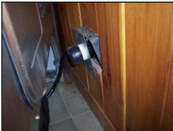
6.3 Picture 1 Stove outlet
