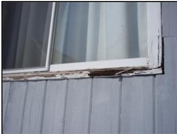
2.4 Picture 1 Water damaged window frame at south side
