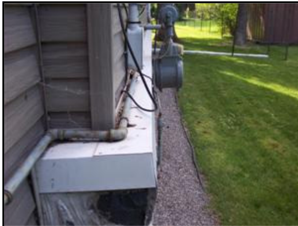
2.0 Picture 1 Flashing at top of foundation wall
