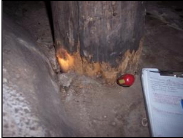
3.2 Picture 1 Wood column near furnace
