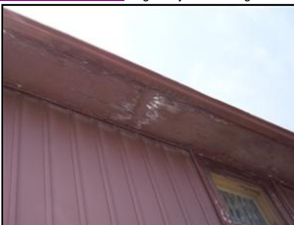
2.2 Picture 1 Water staining at soffits, south side
