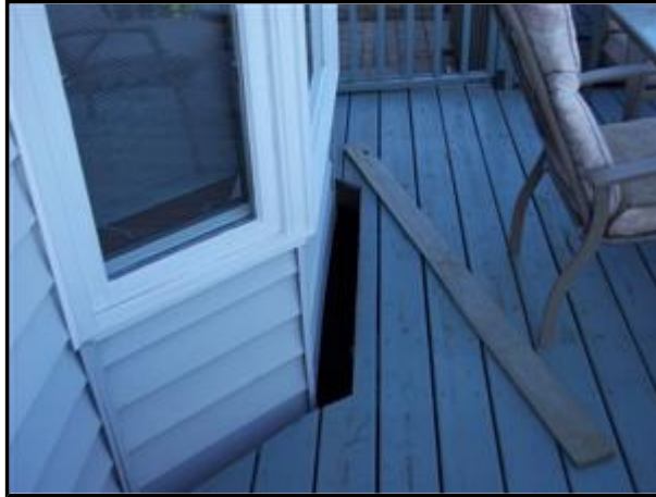
2.5 Picture 1 Gap between house and deck
