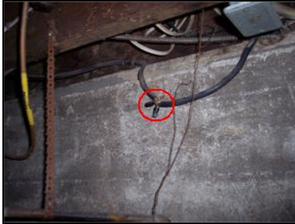
6.3 Picture 2 Unsafe junction at basement (west side)
