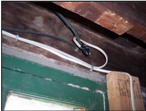
6.3 Picture 3 Improperly terminated circuit above basement east window
