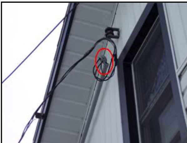
6.0 Picture 1 Missing weather head and unclamped conduit
