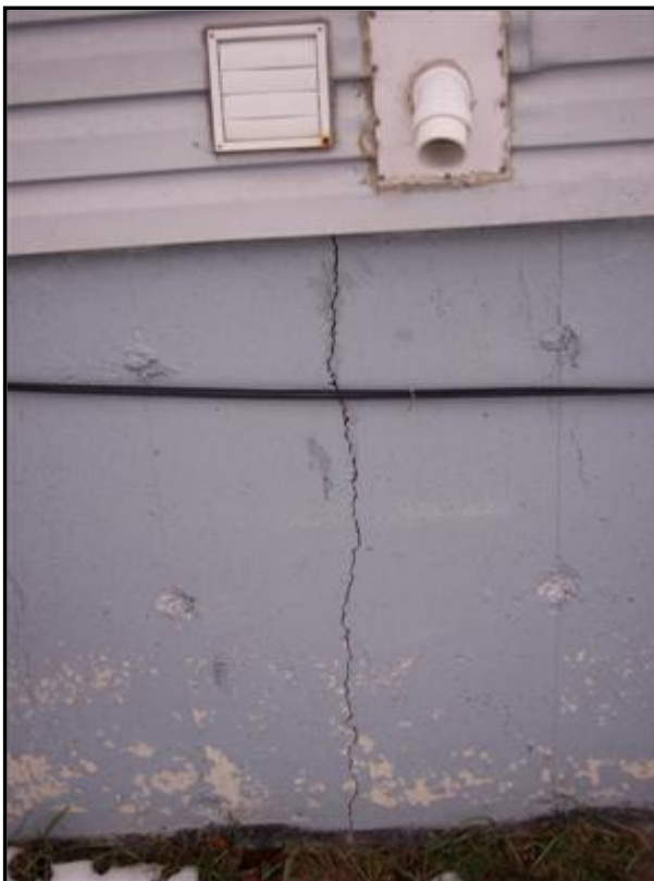
2.1 Picture 1 Crack at south side
